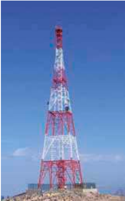
Mast with DF and monitoring antennas and a DF receiver accommodated in an all-weather cabinet on the upper platform.
