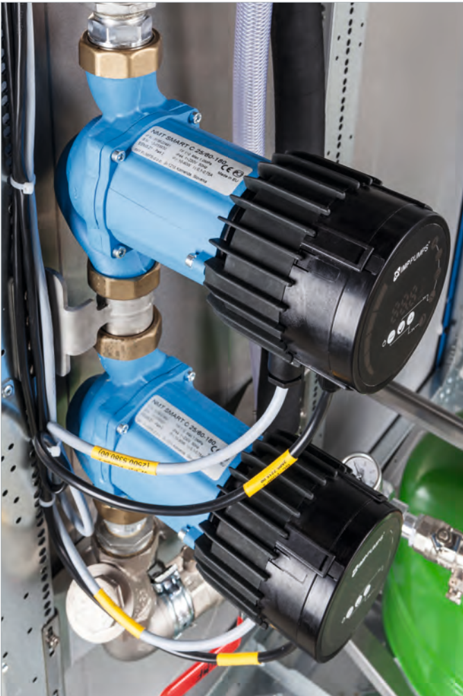
Compact cooling system with redundant pump modules
