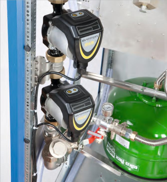
Redundant pump system for multiple transmitter systems.
