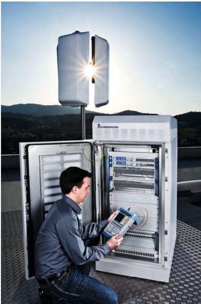
Checking a low-power transmitter by means of the R&S®ETH.
